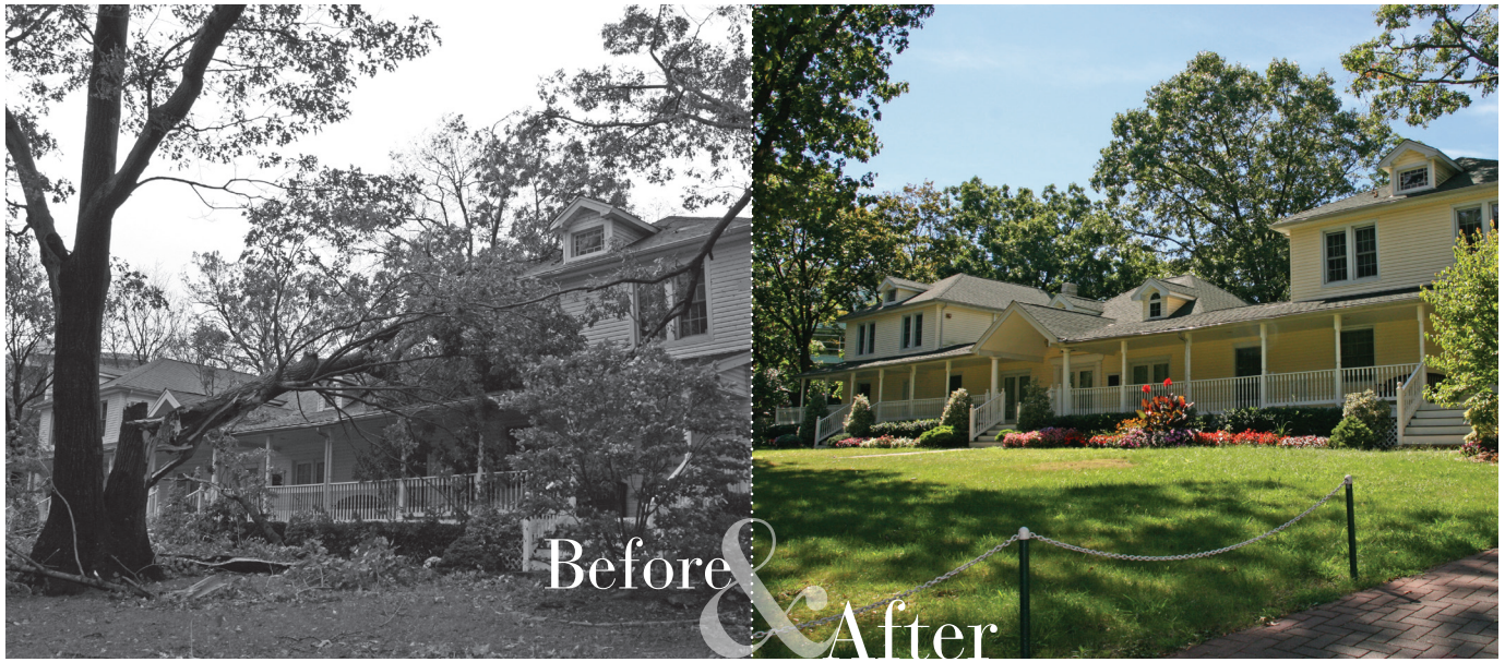
RENEWAL Left: Tree and roof damage on the Pape House, home of Wagner's Office of Admissions, on October 30, 2012. Right: The same view, almost a year later, on September 5, 2013.
