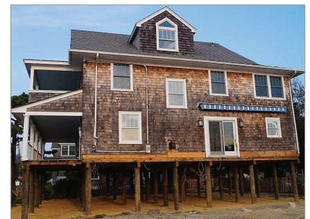
PREPARED The Whites' house in Mantoloking was lifted onto nine-foot pilings.
