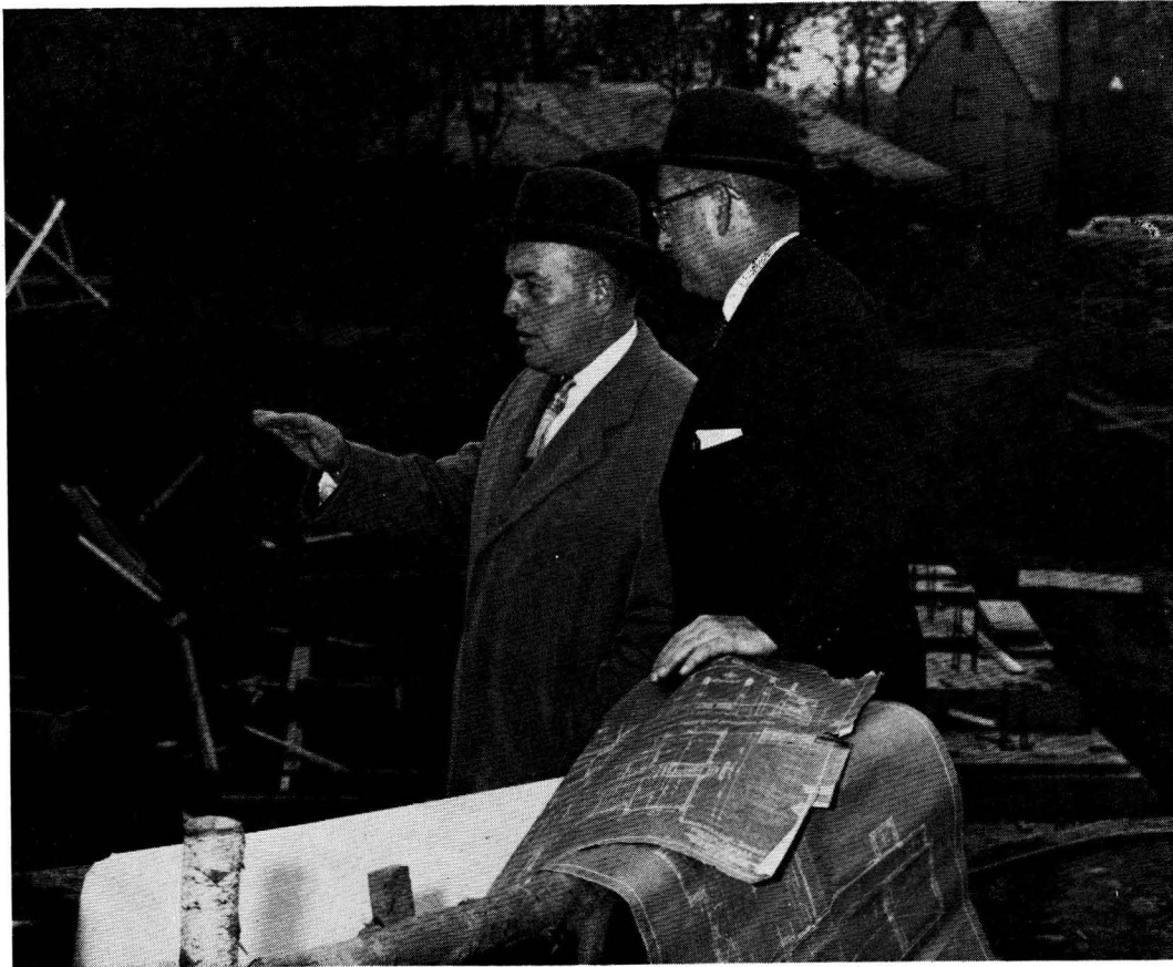
Dr. Delo and John Fisher, Project Manager, survey progress on the new men's dormitory-dining hall.
