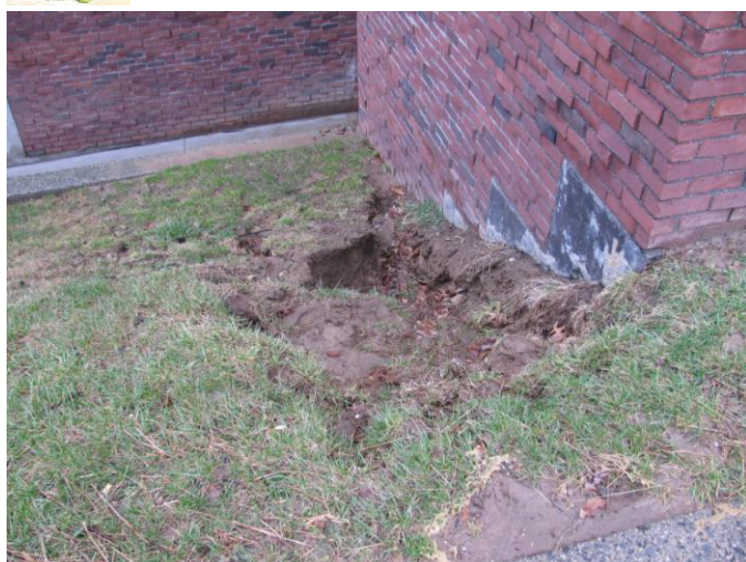
Water damage at the Science Building.
