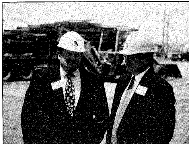
Cameron President Don Davis and Lawton's Goodyear plant manager, Gordon Murdock touring the construction site of the new Sciences Complex at Cameron.
