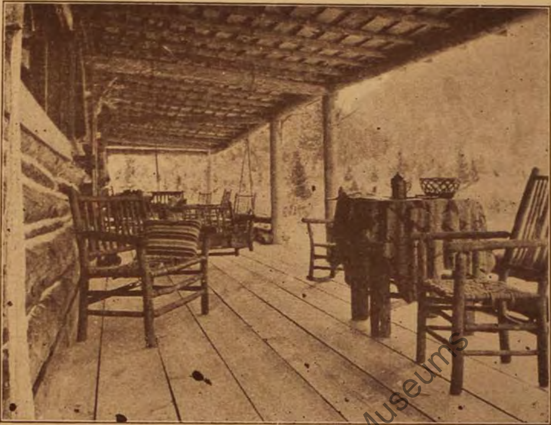
The porch at Hilton
