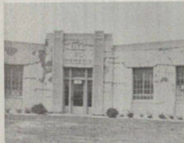
BEFORE—This time-worn City Service Station was a challenge to the Spring Clean-Up Campaign.
