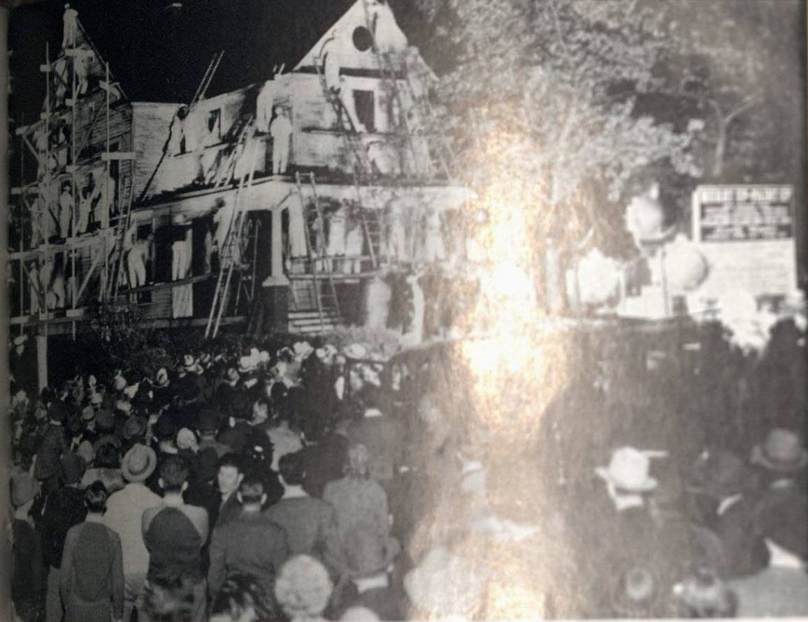
People gather to see a house being renovated during a spectacle promoting Clean Up Week.
