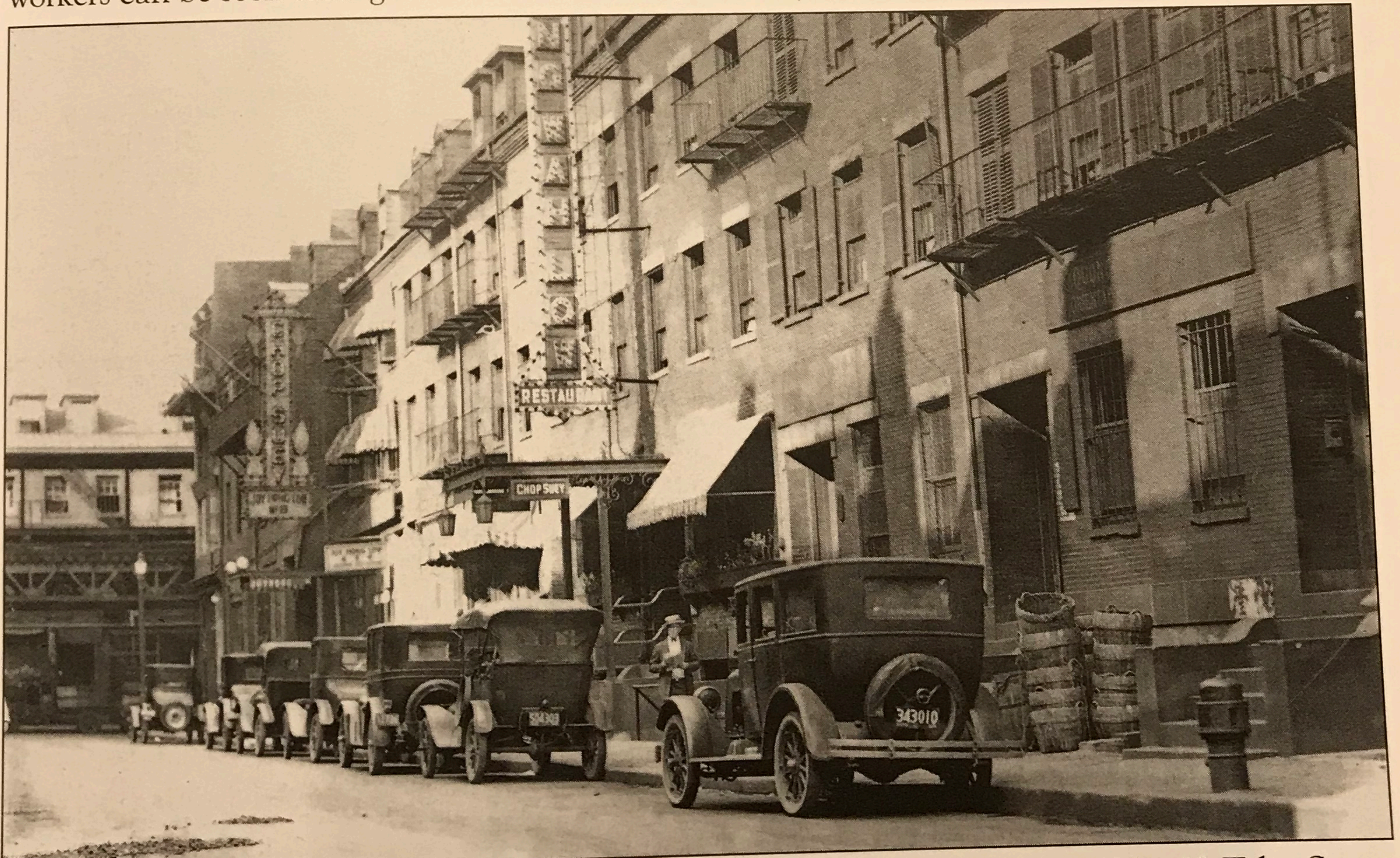
TYLER STREET ON THE RIGHT, c. 1925. The King Wah Low restaurant at No. 12 Tyler Street and the Joy Hong Low restaurant at No. 8 have signage illuminated with light bulbs. The term chop suey became a catchphrase for these and other restaurants to appeal to non-Chinese customers. The street was filled with vehicles along restaurant row. An elevated train track is visible along Beach Street. (Courtesy of International Society.)
