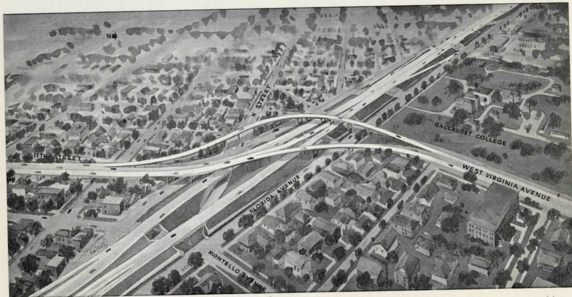
VIEW OF INTERCHANGE BETWEEN EAST AND NORTHEAST SECTIONS — LOOKING WEST
