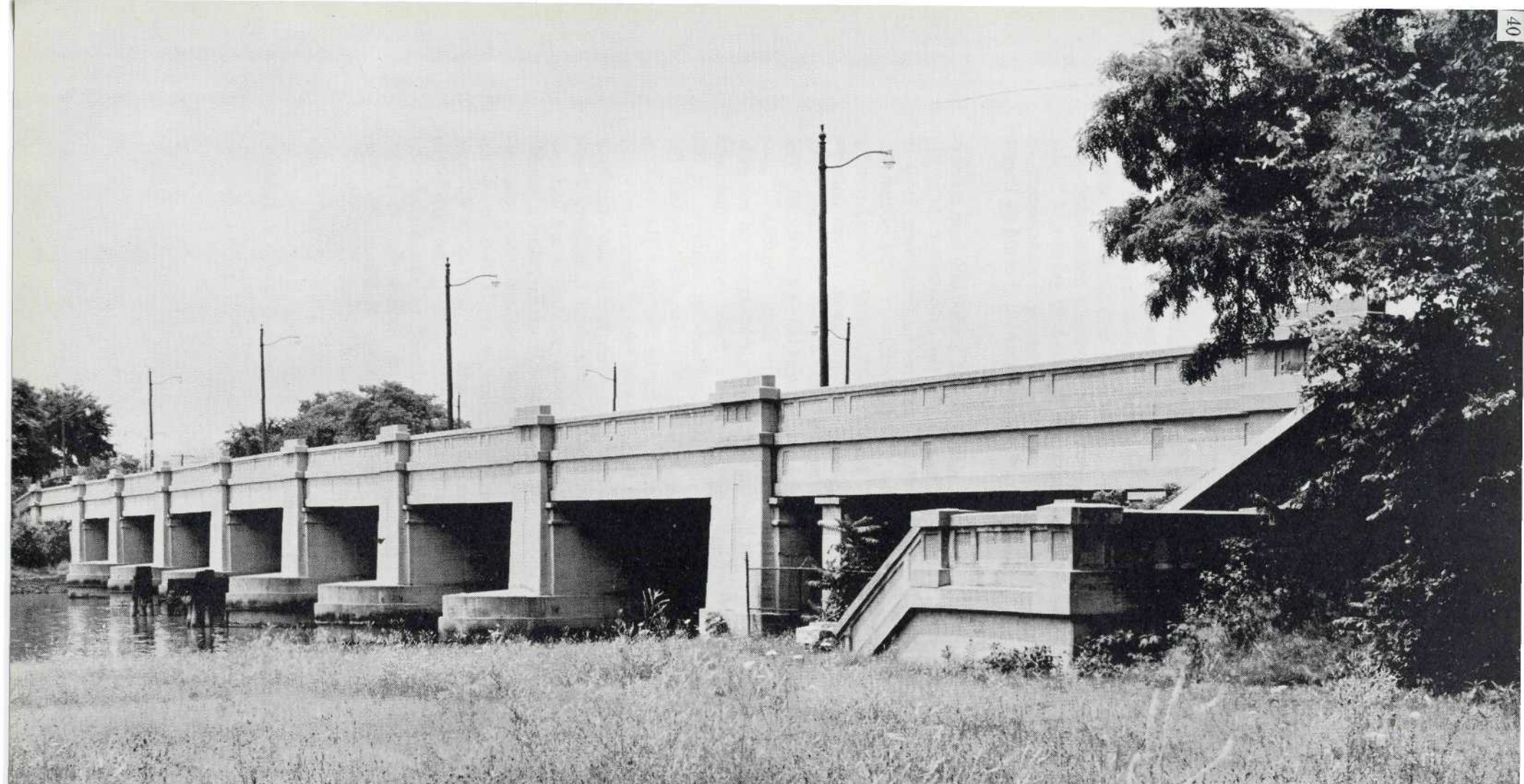
BENNINGS BRIDGE Structural Data Location: Benning Road, N. E., over the Anacostia River Type: steel beams encased in concrete on simple spans Overall length: 586' Width of roadway: 88' Width of sidewalks: 8' each Clearances: (a) river: 40' horizontal—19' vertical (b) highway: 12' vertical (for park roads only) Design load: H20 Special design load: 45-ton trailer (gross) in curb lanes Designers: D. C. Bridge Division Contractors: Kaufman Construction Co., Philadelphia, Pa. Built: 1934 Approximate cost: $356,952
