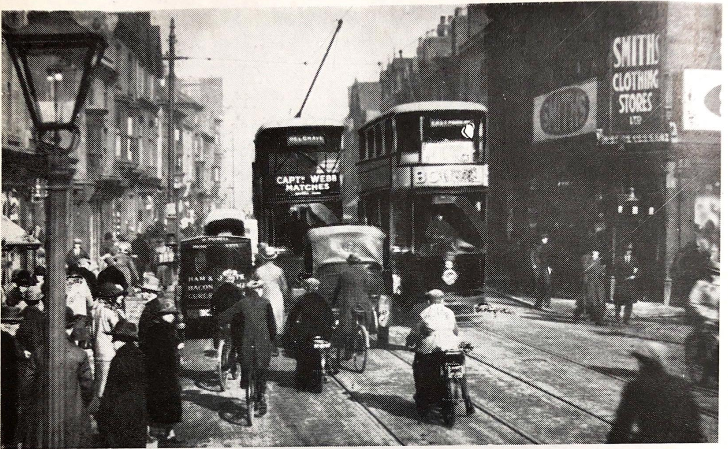
BELGRAVE GATE BEFORE WIDENING
