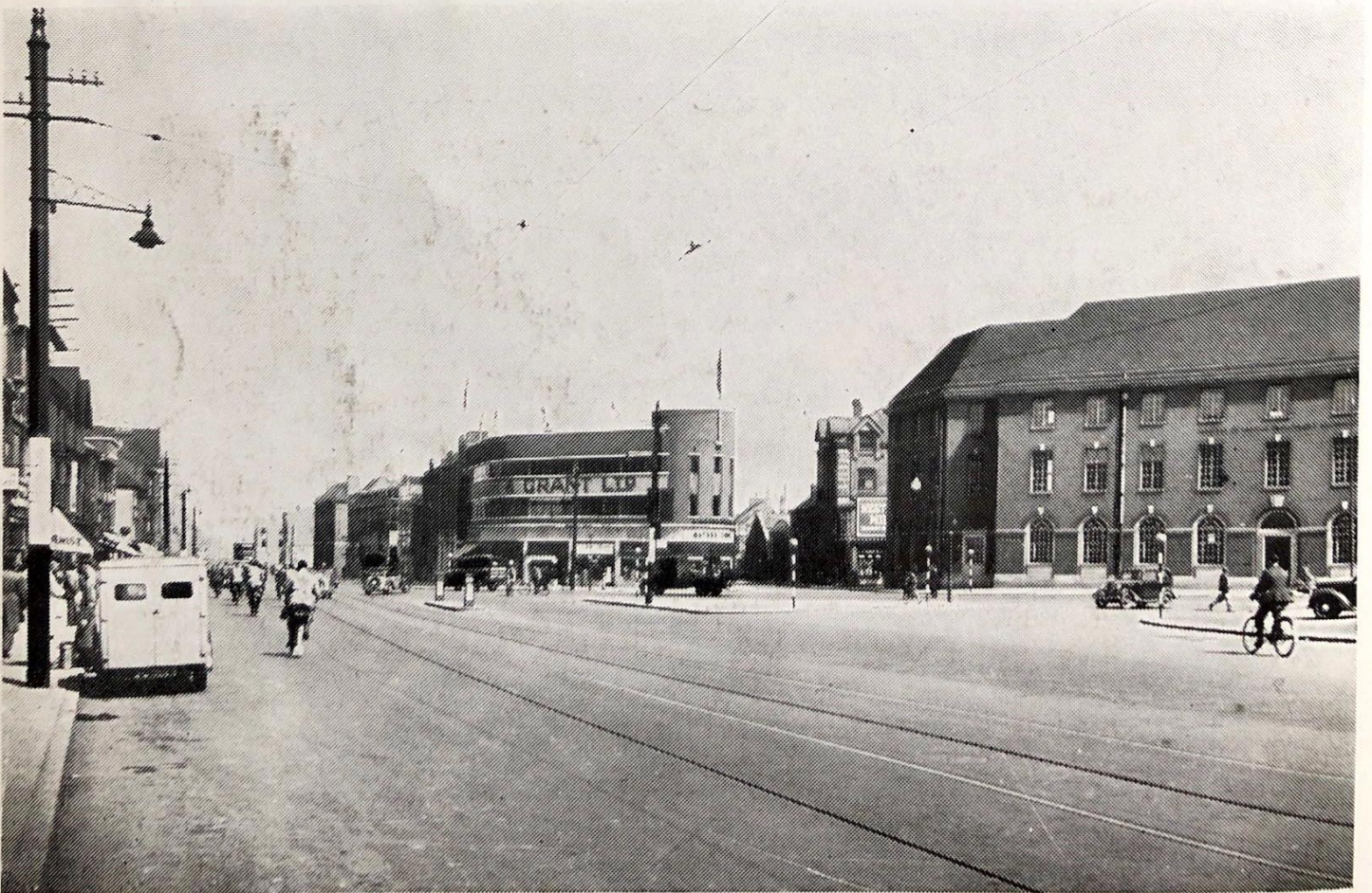
BELGRAVE GATE AFTER WIDENING
