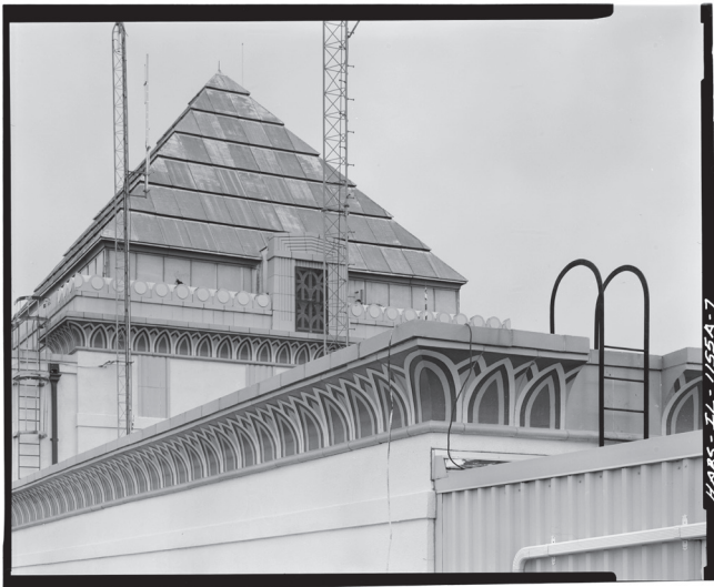
Metal pyramid, cavetto cornice, and Egyptianizing details. Photo Credit: Library of Congress, HABS ILL,100-MAR,1-A--7
