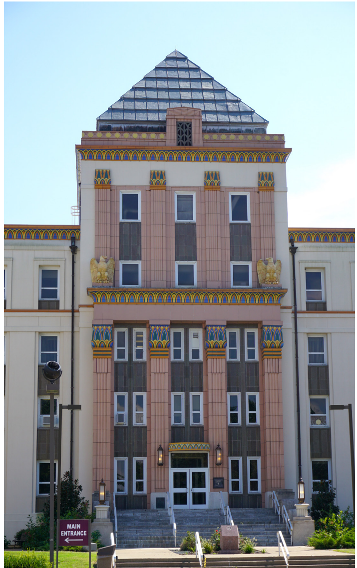
Detail, exterior of main Marion VA Medical Center building. Photo Credit: Stacy Davidson
