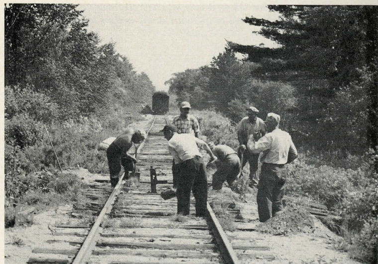
Summer of 1951 found a track gang at work, between Epsom and Short Falls, on part of the road's extensive tie replacing program. Used ties were bought at low cost from the B & M to replace "sleepers," many of which had not been renewed in 25 years. The present year should see the completion of this project
