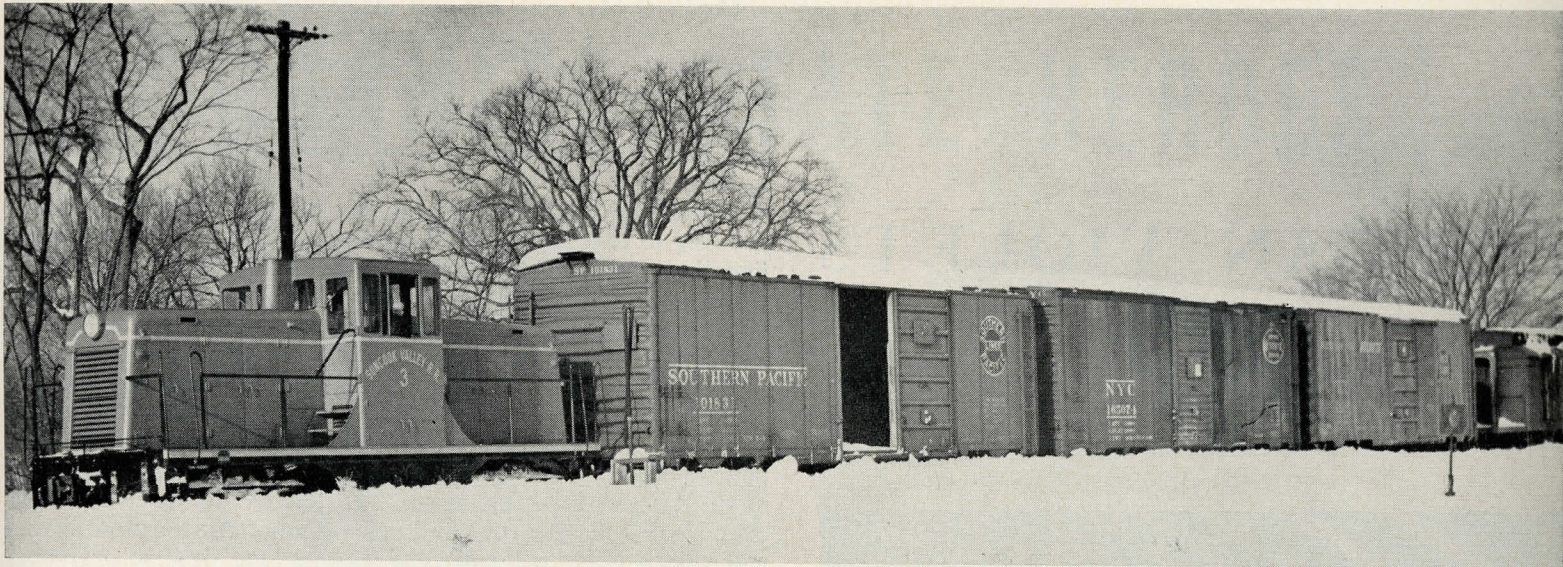
The morning "down" train on the S. V. arrives at Suncook with the cars ahead of, rather than behind, the engine. This unusual situation occurs because of the "switchback" one mile south of the Suncook station, by which the road negotiates the grade to higher ground. After backing into Suncook, the locomotive (No. 3) changes places with the combine, and continues into Concord. On the "up" trip, the procedure is repeated, and the train backs up to the switchback
