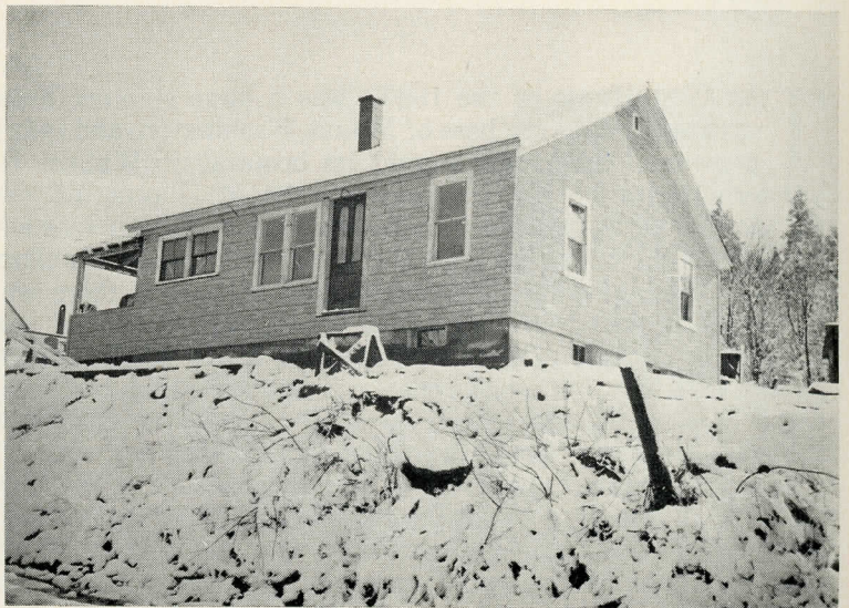
Nearing completion, the Newton home stands on a little hill just outside Groveton, the town that showed it had a heart when it came to the aid of a family unable to help itself. Everyone gave, did what he could, in the way of materials, labor and skills, on a voluntary basis
