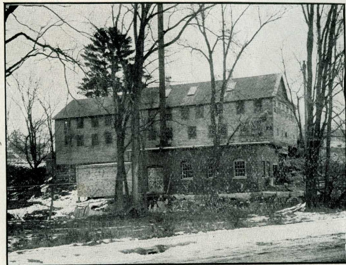
J. F. CLOUTMAN'S ELECTRIC PLANT
