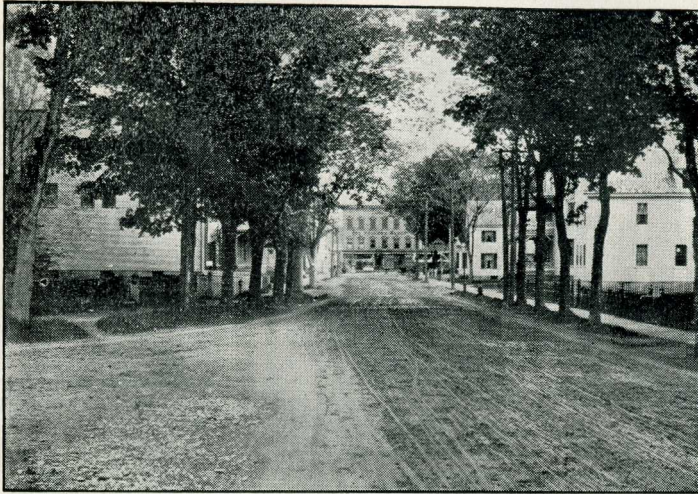
CENTRAL STREET, LOOKING EAST
