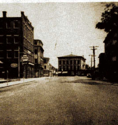
CENTRAL STREET, LOOKING EAST
