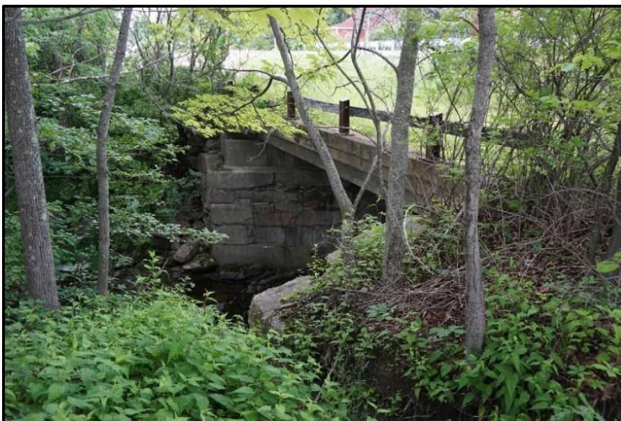
High Street/Flagstone Ave. bridge in 2017 (closed to traffic)
