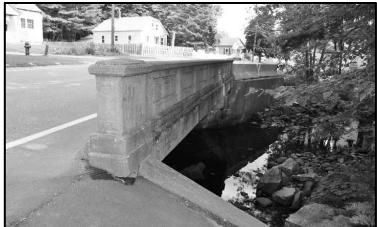
Spring Street Bridge over the Cocheco, 2017
