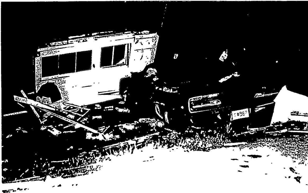
This car ran through the Star Diner last week, carrying with it a section of wall, and equipment from the building.
