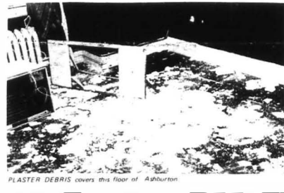
PLASTER DEBRIS covers the floor of Ashburton
