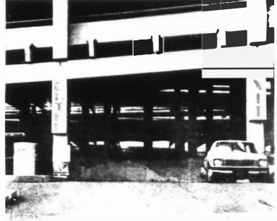
THE GOVERNMENT CENTER GARAGE (above) which was closed this week due to its unsafe condition. A van (left) sits in its hope of a quick re-opening.
