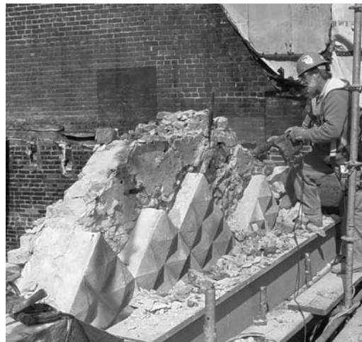
Worker separates stonework from building facade.
