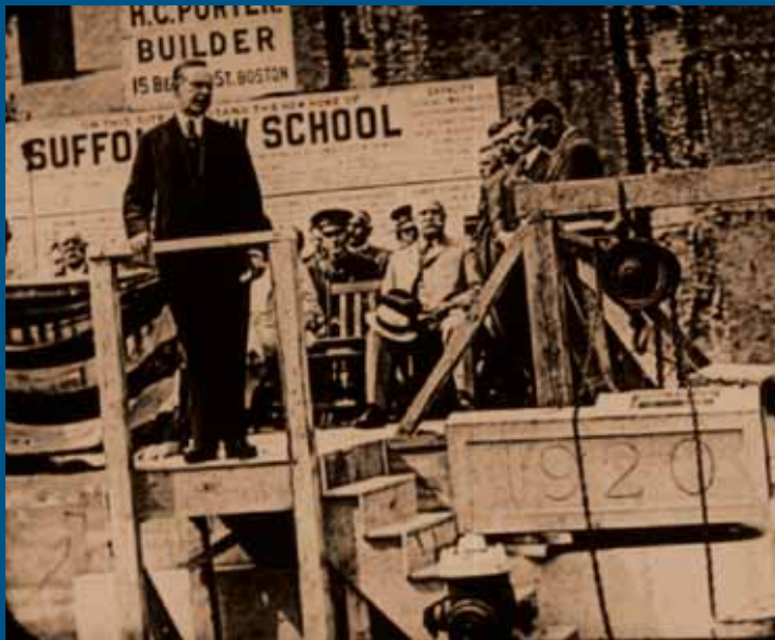
Massachusetts Governor Calvin Coolidge presides over the laying of the cornerstone for what was once the home of Suffolk Law School and what is now the Archer Building, 20 Derne Street, in 1920.
