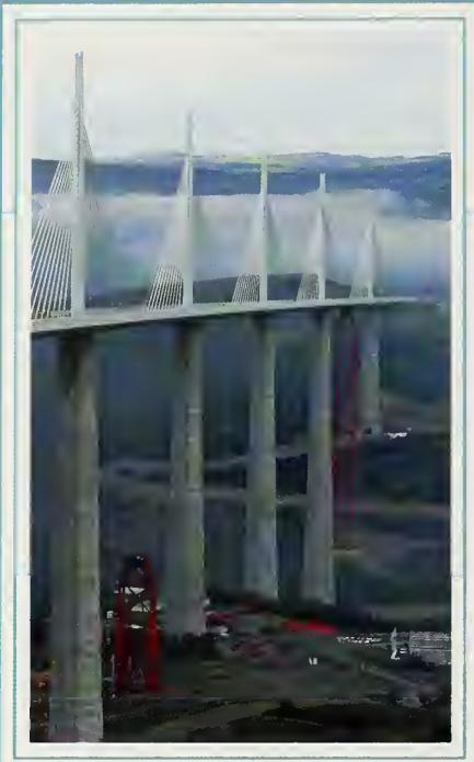
France's 1.6-mile-long Millau bridge extends 1,122 feet above the Tarn Valley, making it the world's tallest roadway span.
