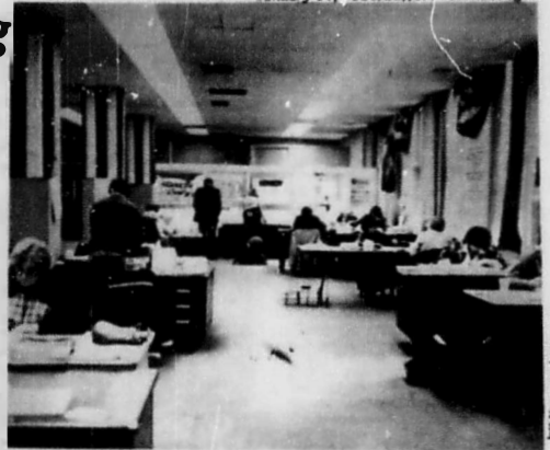
FLOODED WITH WORK, Kennedy campaign workers are striving towards one goal.
