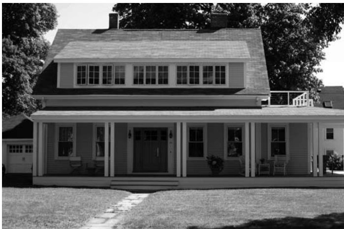
Nancy Hackett’s renovated 1856 house.
