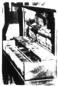
PIANO DAMAGED by Monday fire
