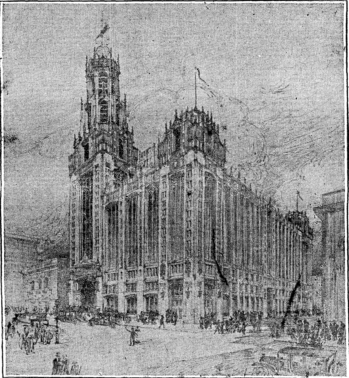
THIS 12-STORY BUILDING, TO COMPRISE A 500-ROOM HOTEL AND A THEATRE TO SEAT 4200 PERSONS, WILL BE ERECTED BY A LOCAL SYNDICATE, ON THE SITE SURROUNDING THE WILBUR THEATRE. THE LAND PURCHASED CONTAINS 55,000 SQUARE FEET, AND IS BOUNDED BY TREMONT, HOLLIS, DILLAWAY, AND DORE STREETS
