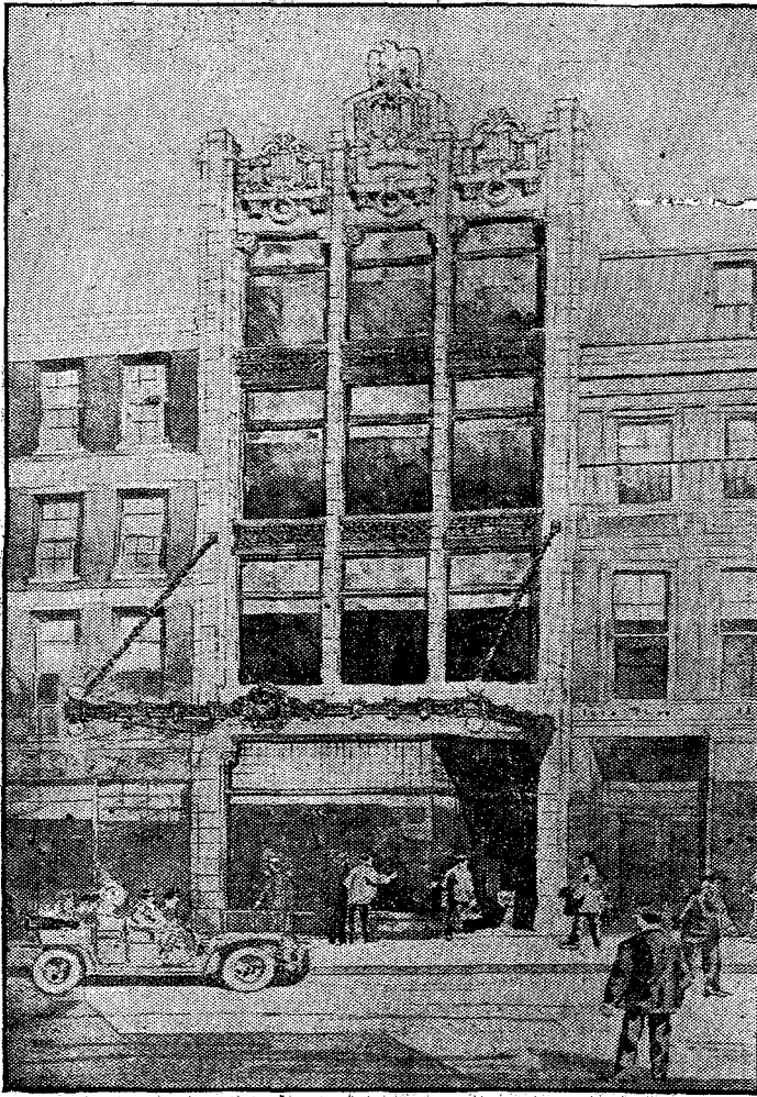
THE WYZANSKI BUILDING, In Process of Construction at 170-172 Washington St.
