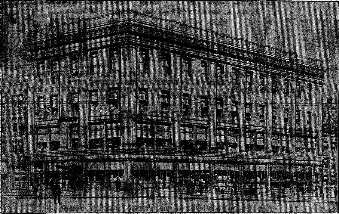
NEW WYZANSKI BUILDING, CORNER GREEN AND CHARDON STS.
