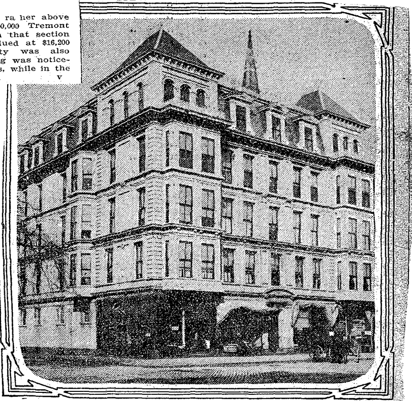
SOUTH END STRUCTURE BOUGHT BY ALVIN D. PUFFER. 565 to 569 Tremont Street.
