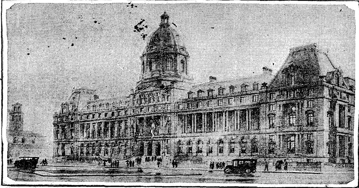
(Study by Cram & Ferguson.) Municipal Building Would Be Part of Group Situated Near Columbus Avenue and Dartmouth Streets.
