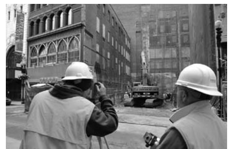
Surveyors at Modern Theatre site (Photo by Renee DeKona)
